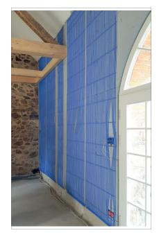
View of a wall section: mat distributor pipes in the screed
